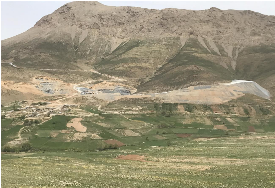
Fig. 7. Mining and road construction activities in the Hashtad Mountain region, illustrating the environmental pressures on the local flora.
